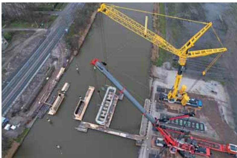
12 Inhijsen prefab kelderbak
