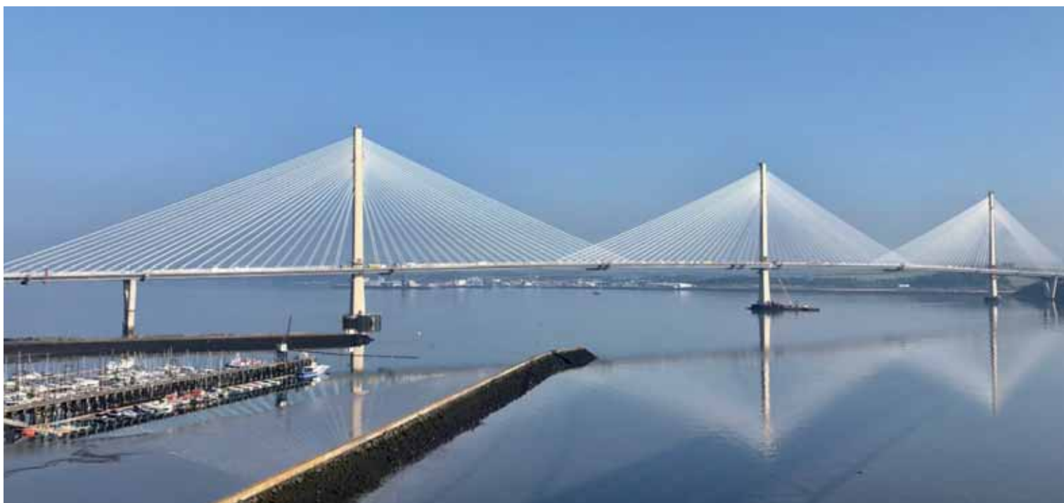
Queensferry Crossing (image: Construction Enquirer)
