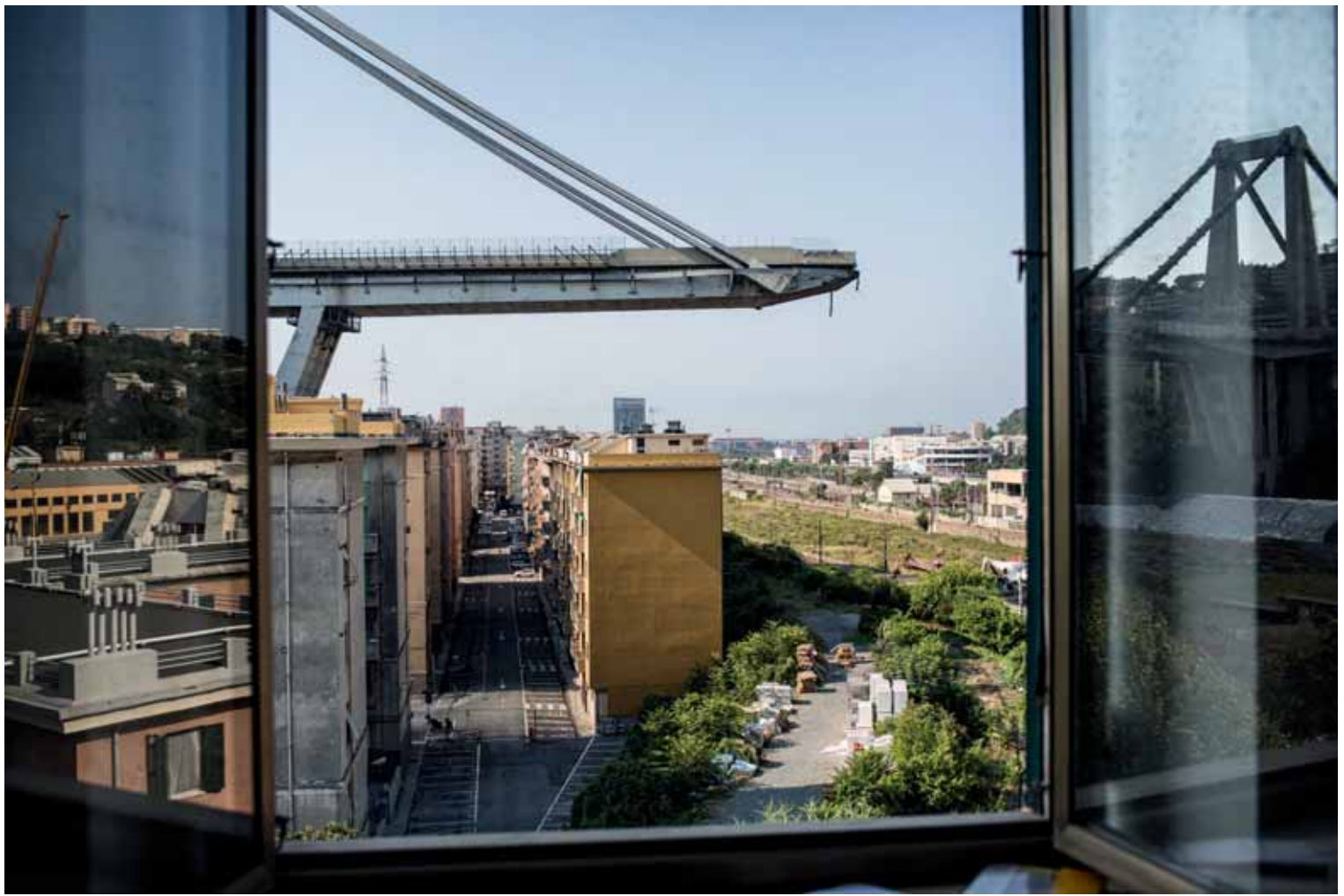
Collapsed Morandi Bridge in Genoa, Italy (image: New York Times)
