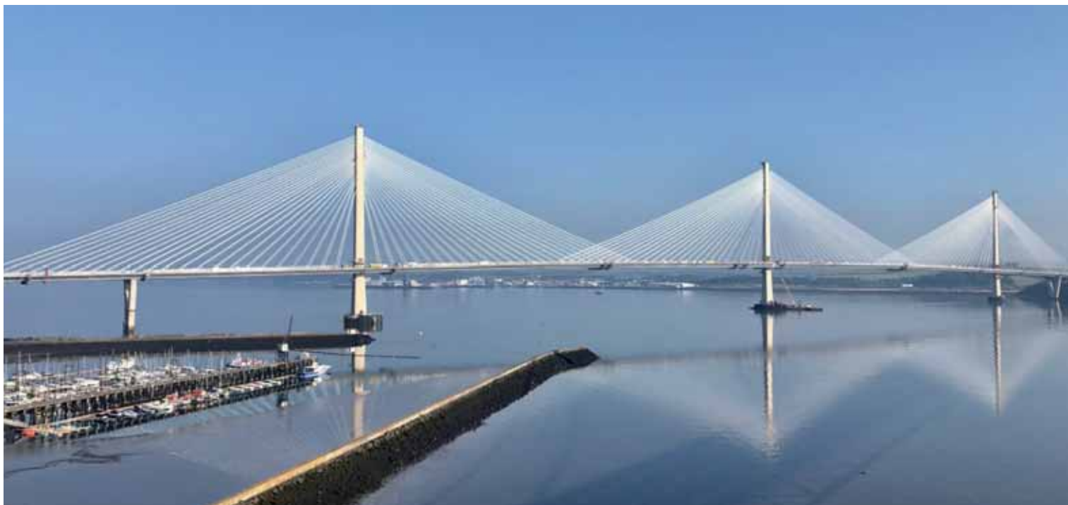
Queensferry Crossing (image: Construction Enquirer)
