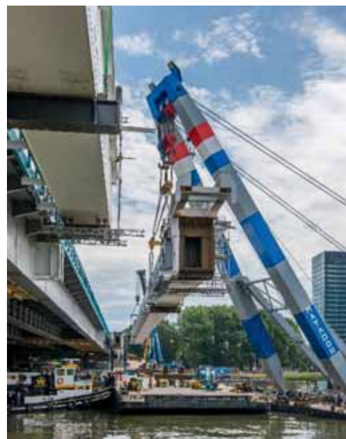
21 Inhangen VSLiggers in Galecopperbrug © Arup
