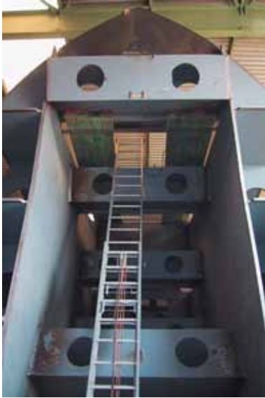
7. Verticale schotten in de pyloon.
