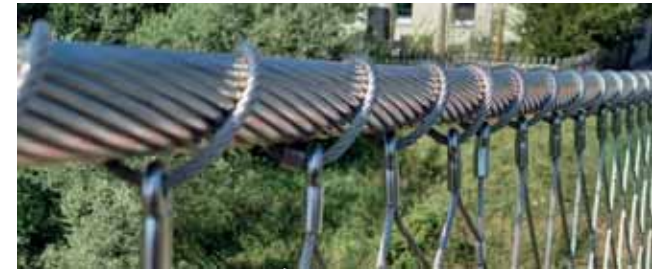
Blocking sleeve on binding rope @ 6th eyelet = approx. 500 mm
