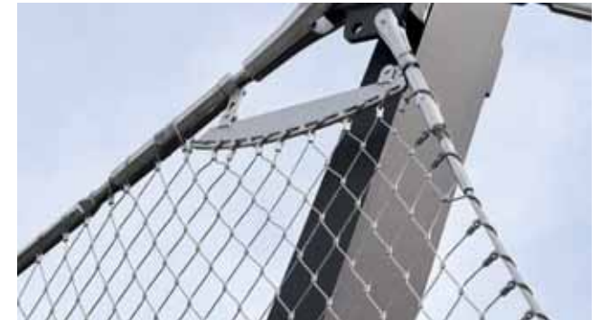
Net corner design, reduction of force peaks
