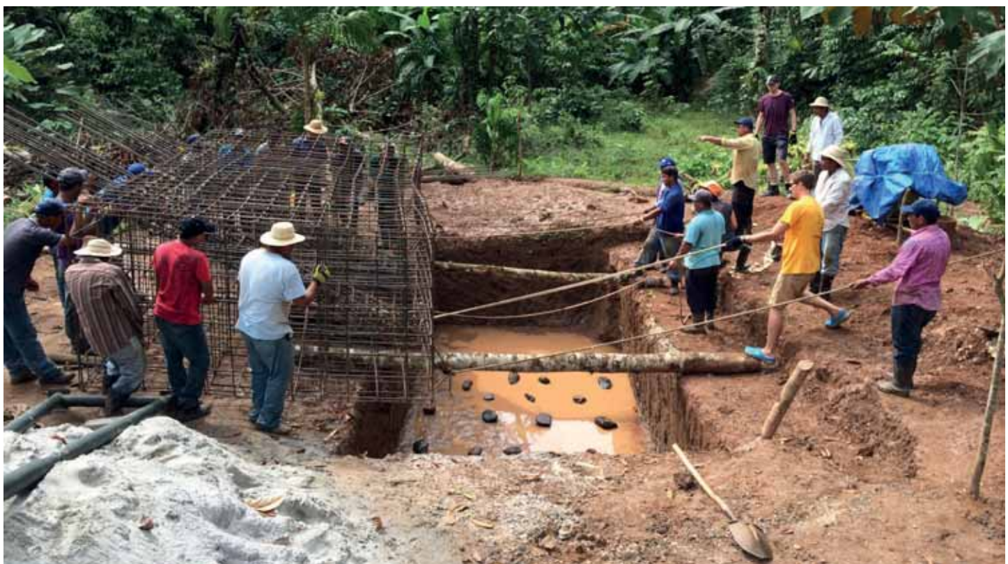
↑ Water in ankerbloksparing
